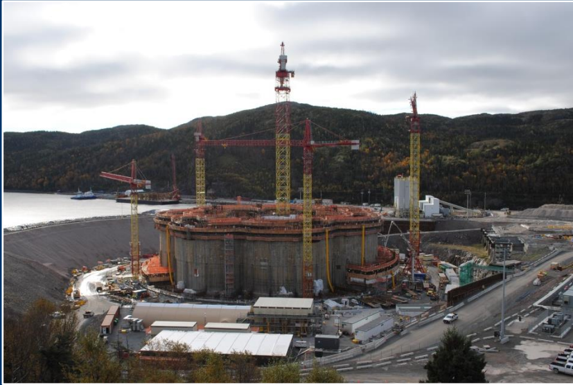
(Photo – Bull Arm Construction Site Oct/2013)
